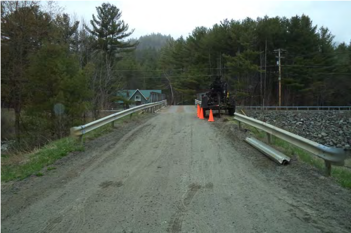
View northwest toward the area of B-1
